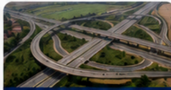
NATIONAL HIGHWAYS AUTHORITY OF INDIA Infrastructure Development
