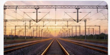
SOUTHERN RAILWAY PROJECTS Infrastructure Development
